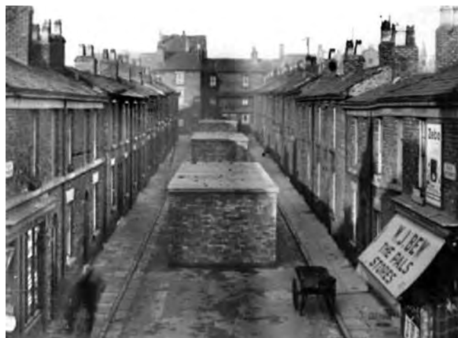
Surface shelters in Fan Street, Liverpool
